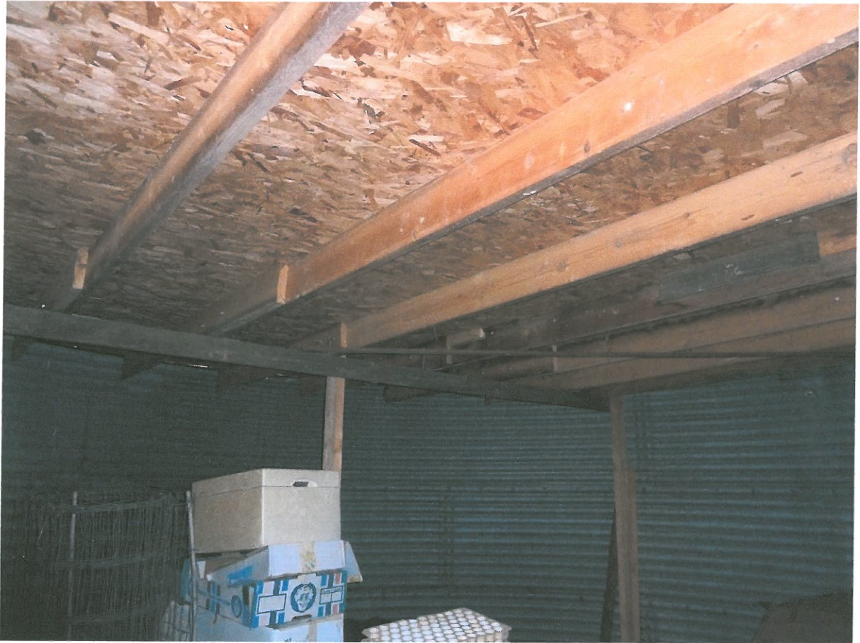
Photo 3. Solid roof construction
