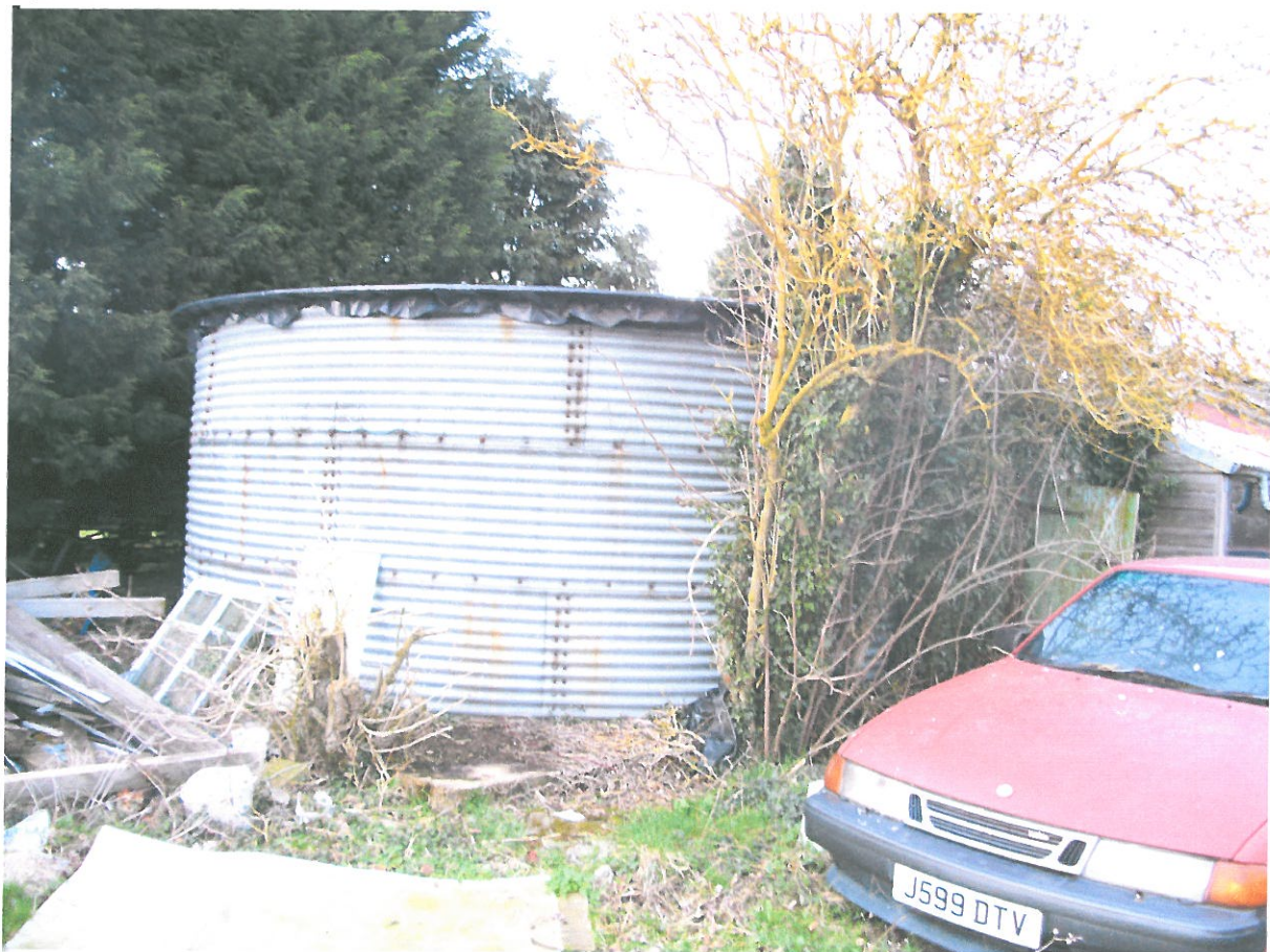
Photo 7. External view of converted water tank.
