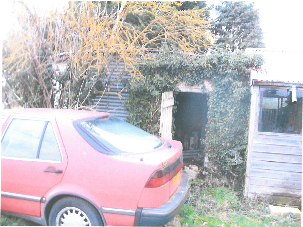
Photo 6. View showing pump house with doorway cut into former water tank.
